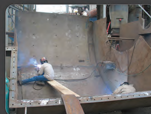
Replaceable ID Fan Housing Liners
